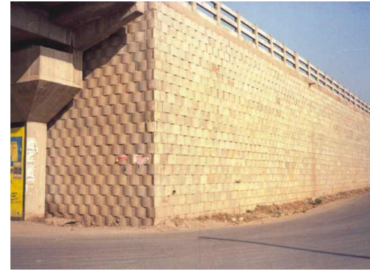
Roads RE Wall
