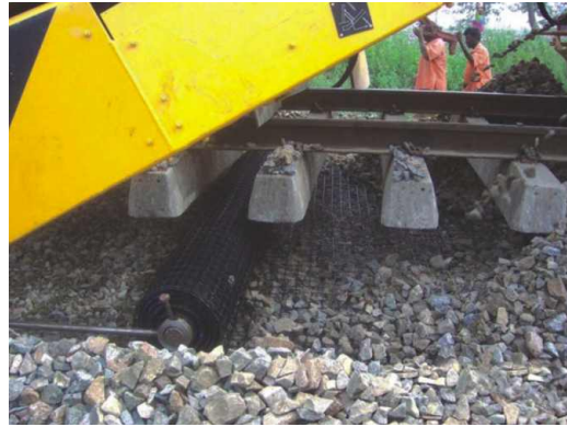
Railway Track Bed Stabilization
