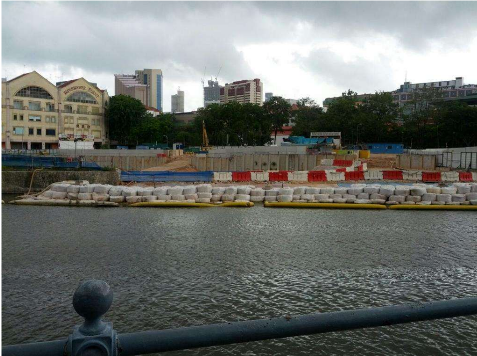
Singapore river bank protection using Geo-containers, Singapore
