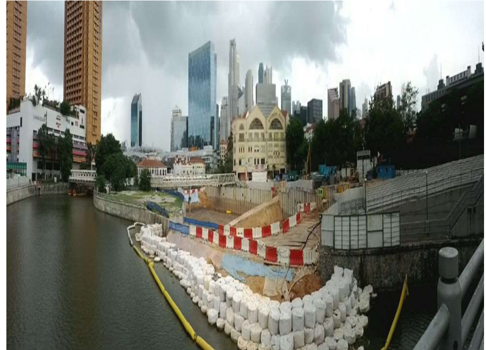
Singapore river bank protection using Geo-containers, Singapore
