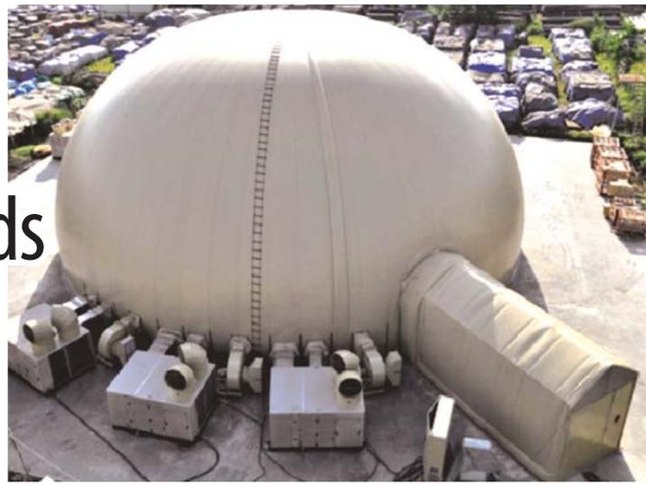
**RADOME, a structural, weatherproof enclosures used to protect an antenna**
